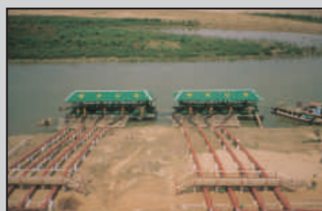
Banhe pumping station, Lao PDR
