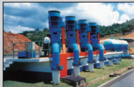
Langkawi water supply project, Malaysia
