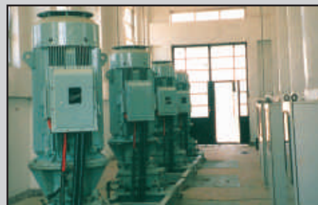
Irrigation Project at Wadi Sheeh, Egypt
